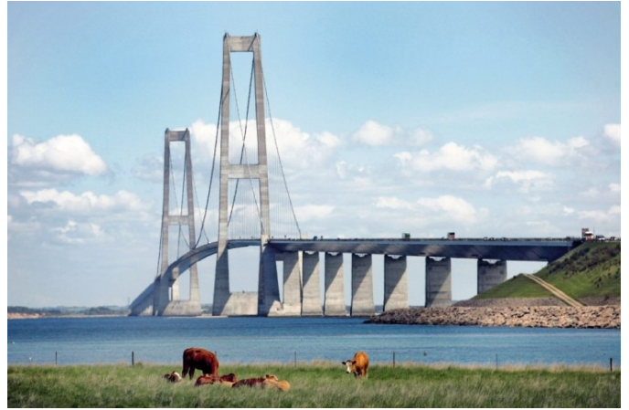
Figure 7. LM-S installed at Great Belt Bridge, Denmark
