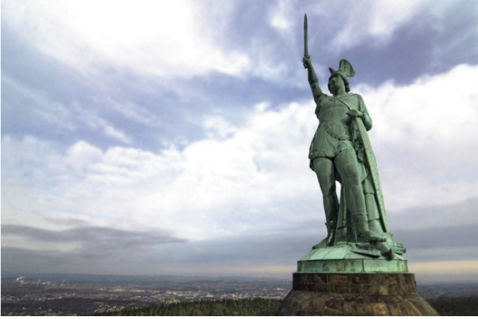
Figure 5. LM-S installed at Herman the German Statue, Detmold, Germany
