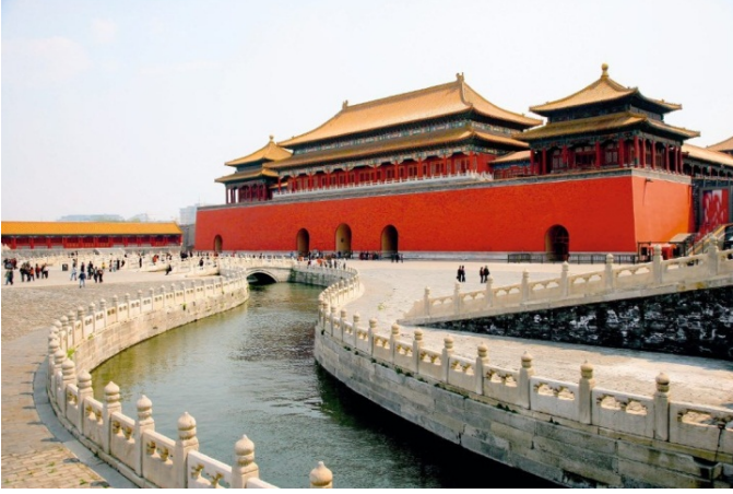
Figure 9. LM-S installed at Women Gate, Forbidden City, Beijing, China
