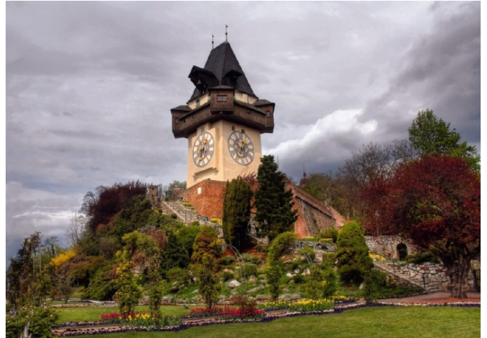
Figure 8. LM-S installed at Clock Tower, Graz, Austria
