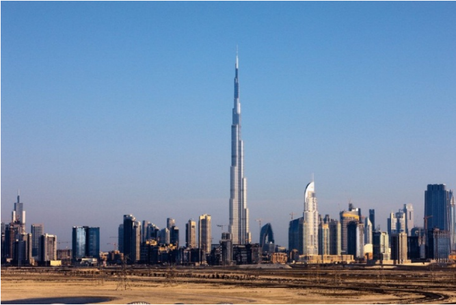
Figure 6. LM-S installed at Burj Khalifa, Dubai, United Arab Emirates
